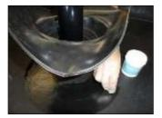
2) Once in position clamp the seal to the pipe with the supplied metal clamp and mark around the base of the seal to give a line to prime up to. Pull pipe seal upwards on pipe to expose the membrane and apply ClassicBond EPDM Primer to the EPDM deck membrane
