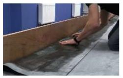
2) Once the adhesive has become touch dry with no wet puddles, mate the two surfaces together. Leaving no voids between the ClassicBond membrane and the receiving surface
