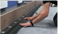
3) Once the primer is dry remove the protective strip from the PS tape on the RUSS. Lay the primed membrane into the PS tape with no wrinkles or air gaps and smooth in by hand then roll with hand roller.
