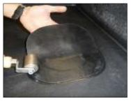
2) Apply the Uncured PS tape to the primed area. Once fitted cut a small section from the centre of the tape out to expose the outlet opening and press the remainding tape down into the outlet. Roll the entire flashing with hand roller.
