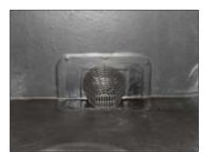
3) Once the second section of tape is installed, complete by inserting the leaf grate into the outlet.
