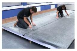
3) Lay the top membrane onto the Seam Tape. Pull away the poly backing from the tape at a 45° degree angle to the seam. While removing the poly backing, draw your hand across the seam, from the back to the leading edge. Roll the seam at right angles to the seam direction, not along it.
