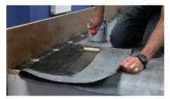
4) Once bonded to the RUSS finish the upstand by using Bonding Adhesive to the remainder of the RUSS, upstand and membrane.
