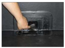
2) Install Uncured PS tape to the outlet. This should be large enough to join onto the membrane by a minimum of 50mm. Cut a small square out of the middle of the tape and mould the tape into the outlet pipe by 25mm. Cut a second section of Uncured PS tape 100mm wide. This will be inserted into the outlet pipe to reinforce and lengthen the tape that was turned into the pipe by 25mm. Apply
