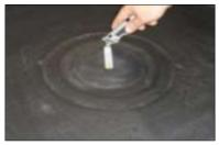
1) Fit the outlet into the roof before installing the membrane; ensure the outlet has the yellow protective cap installed. Install the ClassicBond EPDM membrane to the roof and over the outlet, place cutting guide over the pin and cut round the circular plate.
