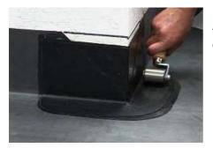
4) Work the tape onto the deck around the corner and smooth out and roll the entire flashing with hand roller.
