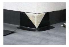
2) Apply ClassicBond Primer to the marked area to be flashed and allow to dry. The area must be clean and dry before application of primer, apply primer to membrane and to upstand substrate. ClassicBond Primer must be allowed to dry before application of tapes.
