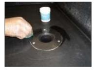
1) Cut the outlet flange back to leave a min. 50mm head and cut the membrane back to meet the perimeter of the outlet head. Secure the outlet into the decking and apply ClassicBond Primer to the head of the outlet and to the EPDM membrane.
