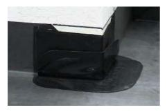
3) Start installing the tape from the top point. Work the tape down upstands first and into the bottom angle change.
