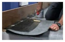
1) Apply the Bonding adhesive to the side of the RUSS or exposed decking. Also apply the Bonding adhesive to the relevant upstand termination or step down and to the back side of the ClassicBond membrane.
