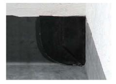
3) Roll the taped area with hand roller once installed.
