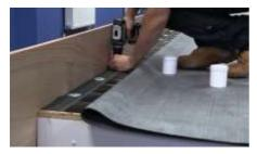
1) Mechanically fasten the RUSS horizontally into the decking or into the upstand with the PS section being to the inside of the roof.
