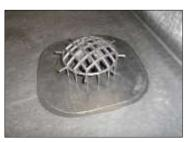
3) Finally install the leaf grate to complete the 68mm flat roof outlet.
