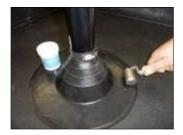
3) Pull pipe seal back down over pipe and into position. Remove poly backing from the tape and with hand pressure press tape onto primed area. Roll splice area with a hand roller
