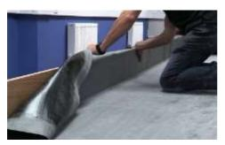
3) Applying positive pressure to the membrane work the membrane up the upstand to the desired height. These areas should be rolled to achieve a strong bond between membrane and substrate.
