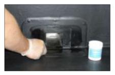
1) Install outlet into parapet wall before installing EPDM membrane. Install the ClassicBond EPDM membrane over the outlet with ClassicBond Bonding Adhesive. Cut the EPDM membrane away from outlet opening by 50mm. Apply ClassicBond Primer to the membrane, outlet face and into the outlet pipe.
