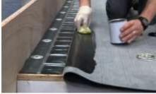
2) Apply ClassicBond Primer to the area on the underside of the EPDM membrane that will come into contact with the 75mm PS tape on the RUSS.
